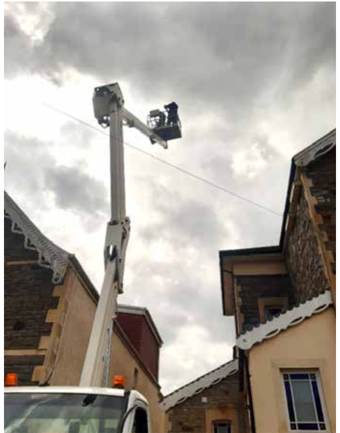
Two double boxes just installed on the house on the right. Toby and Justin decide to check the swift's eye view, which you can see below
