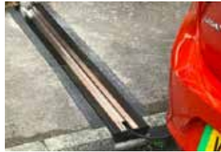
A pavement gully
